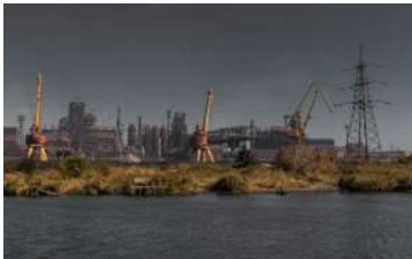
Figure 248: Azovstal iron and steel works (Image Chad Nagle under the CC-BY 2.0 license)
