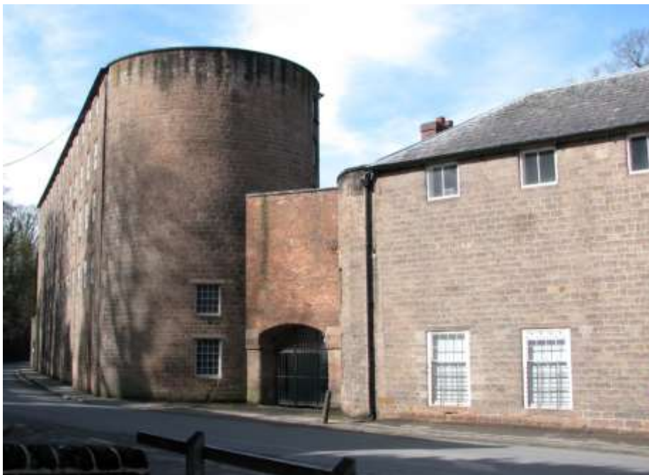
Figure 281: The outside of the mill (seen from the mill manager's house) looks more like a fortress. (Image Roser)
