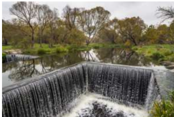
Figure 236: Water flowing over Dam (Image FedBul with permission)
