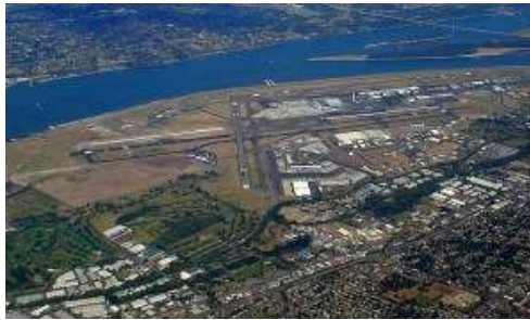
Figure 291: Portland International Airport (Image mike teague under the CC-BY-SA 3.0 license)
